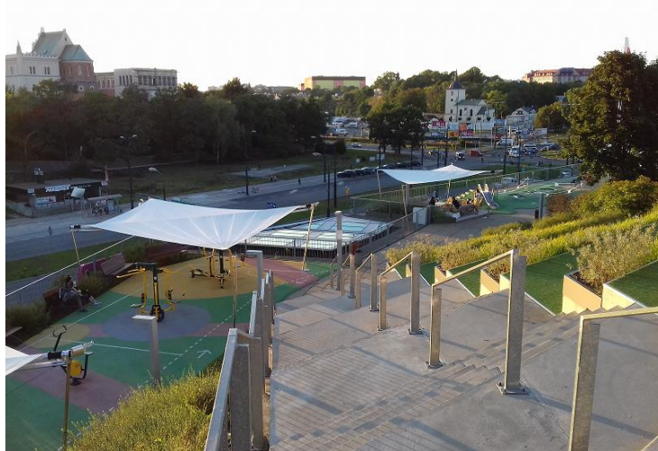
Fig. 4. The roof intense– recreational space, the panorama of the city, Lublin 2022 (photo: M.Tubielewicz-Michalczuk)
